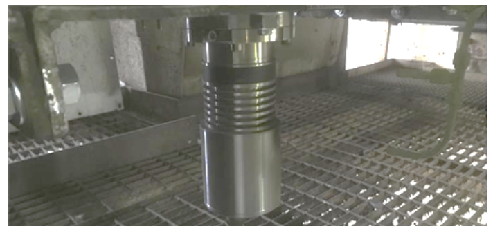
Figure 3: Hydro-Mix HT Installed
